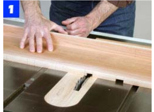
After cutting the 1 x 8 lattice stock to length, lay out the half-lap joint notches and cut them with a dado blade.
