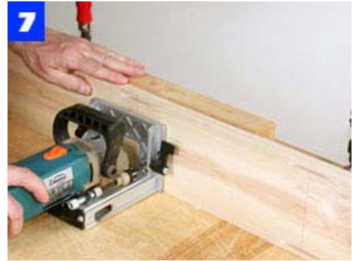
Lay out plate joints in the post parts and cut the slots. The plates keep the pieces aligned during assembly.
